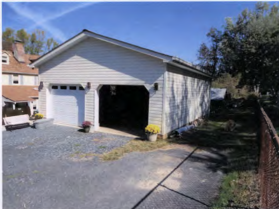
Figure 10 – 11919 Jericho Road, Neighbor directly to rear, Existing 0 foot setback to Property Line along 10 Alley
