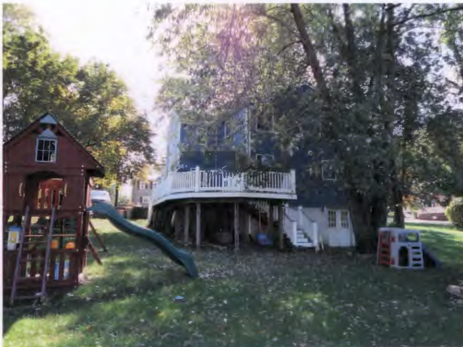
Figure 2 - Existing House Rear View Looking Towards Location of Proposed Addition
