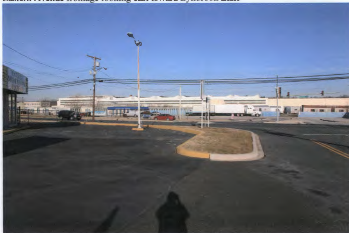
Lynbrook Lane frontage looking north toward Eastern Avenue
