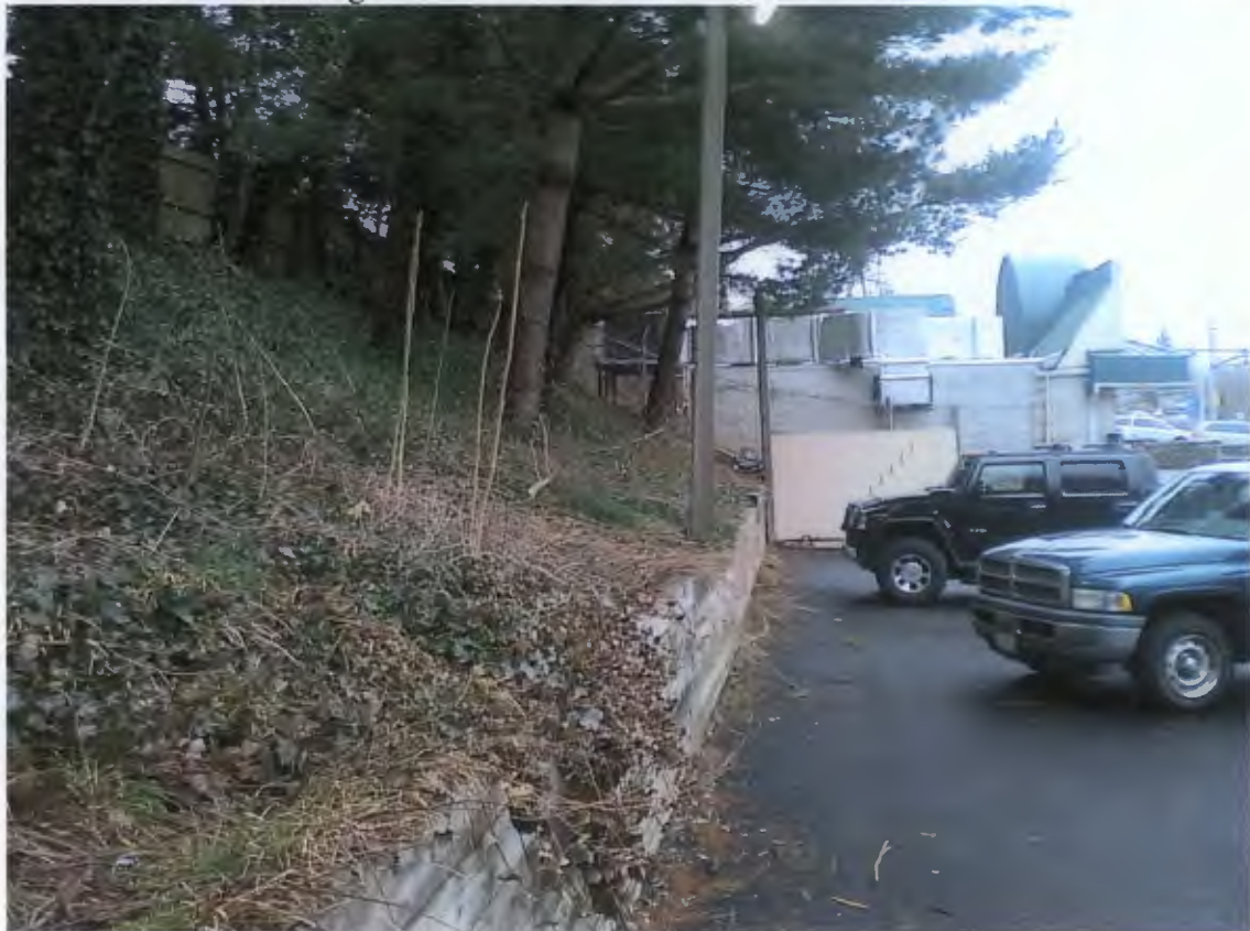
Retaining wall and slope along rear of the property
