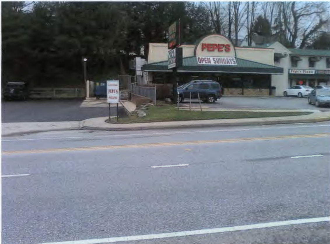
Area between properties with retaining wall to make up grade difference.
