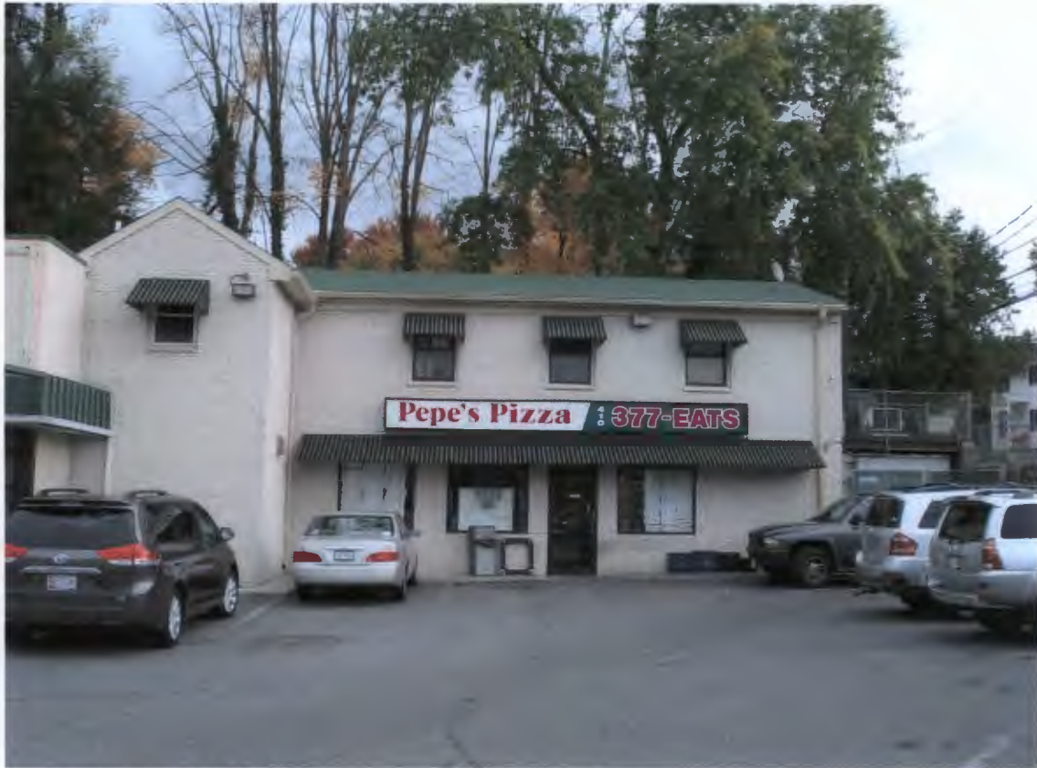
From Falls Road existing area where addition will be constructed
