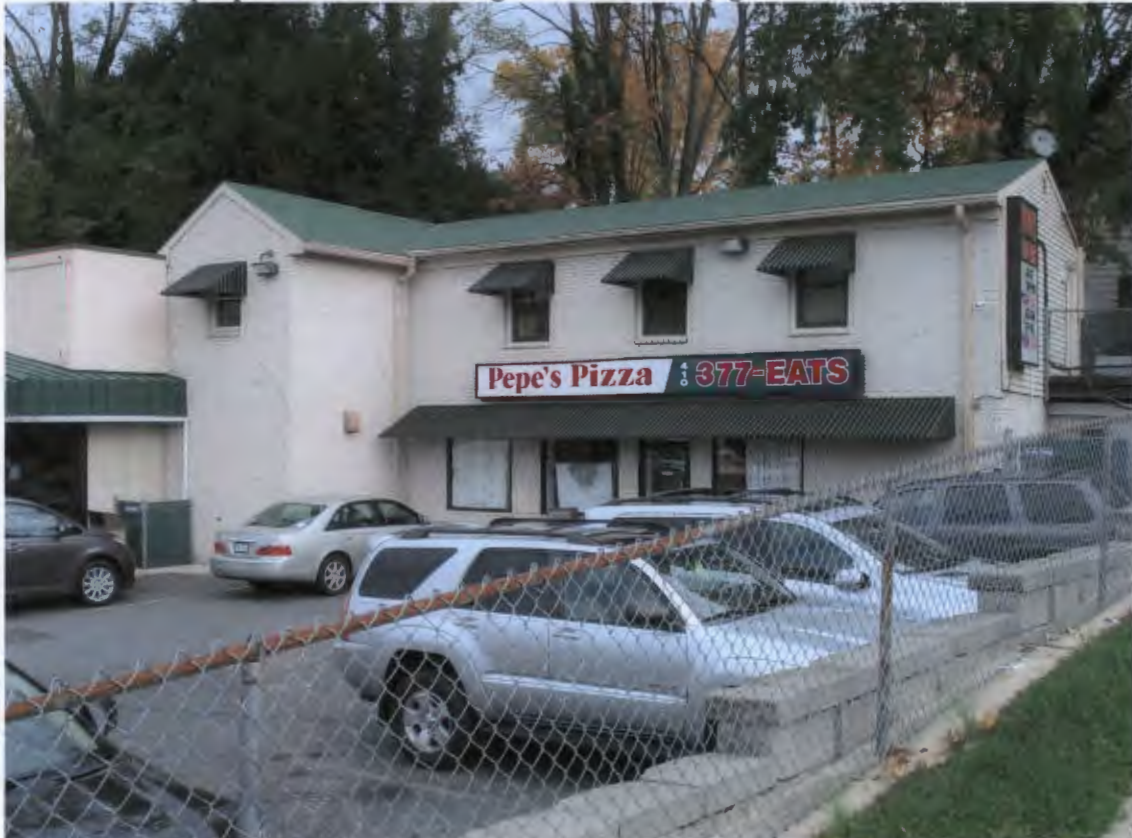
Area where addition will be constructed to square off building
