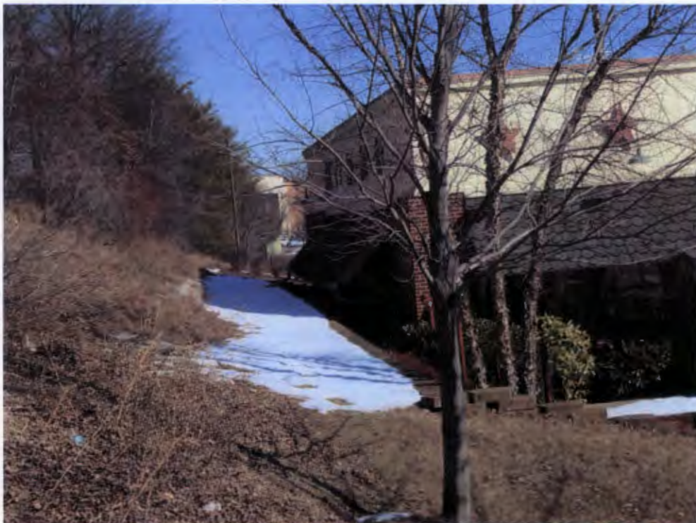
Slope to rear of building looking Northeast
