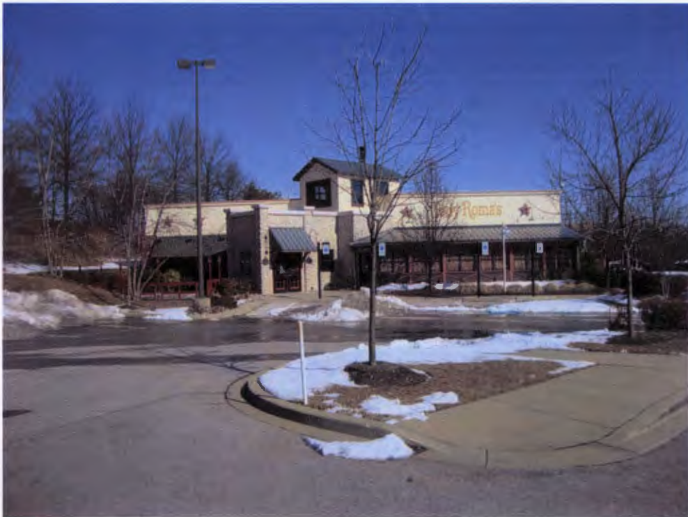
Site from Restaurant Park Drive North, looking Northeast
