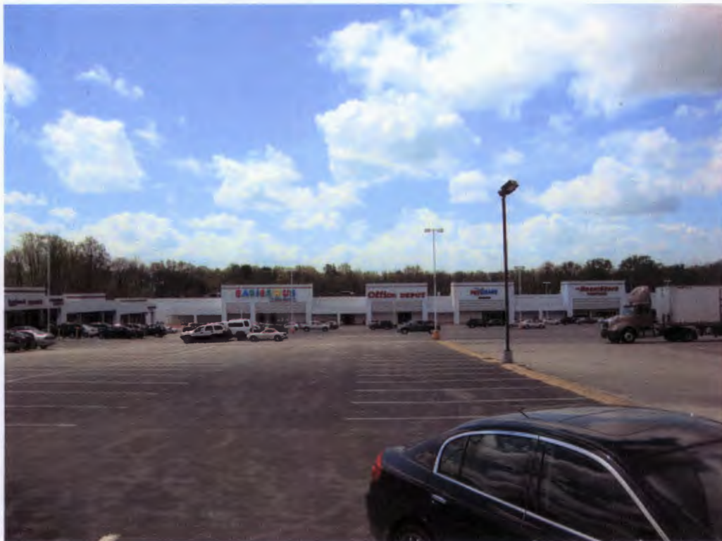
View of remainder of Shopping Center from Baltimore National Pike
