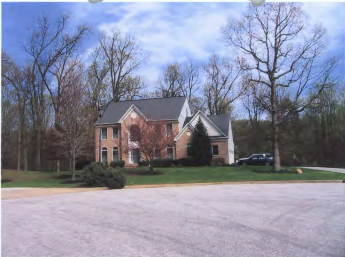
PHOTO # 1 11 Grace Ridge Court From Cul-de-Sac
