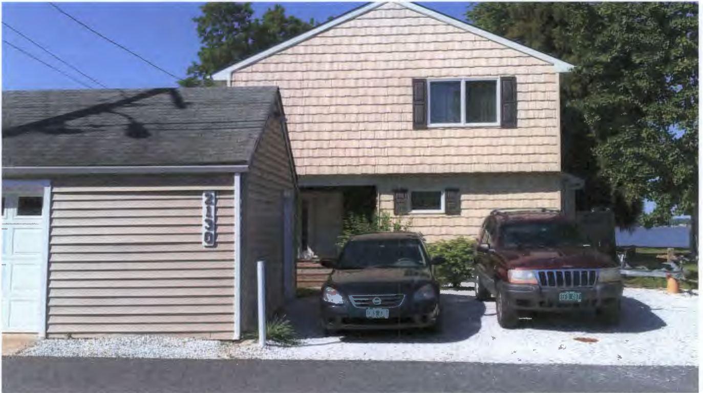
STANDING ACROSS STREET FACING SOUTH TOWARDS PROPERTY
