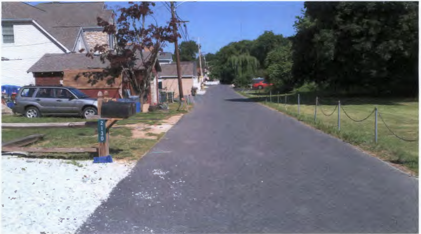
STANDING IN RIVERVIEW ROAD FACING WEST DOWN STREET
