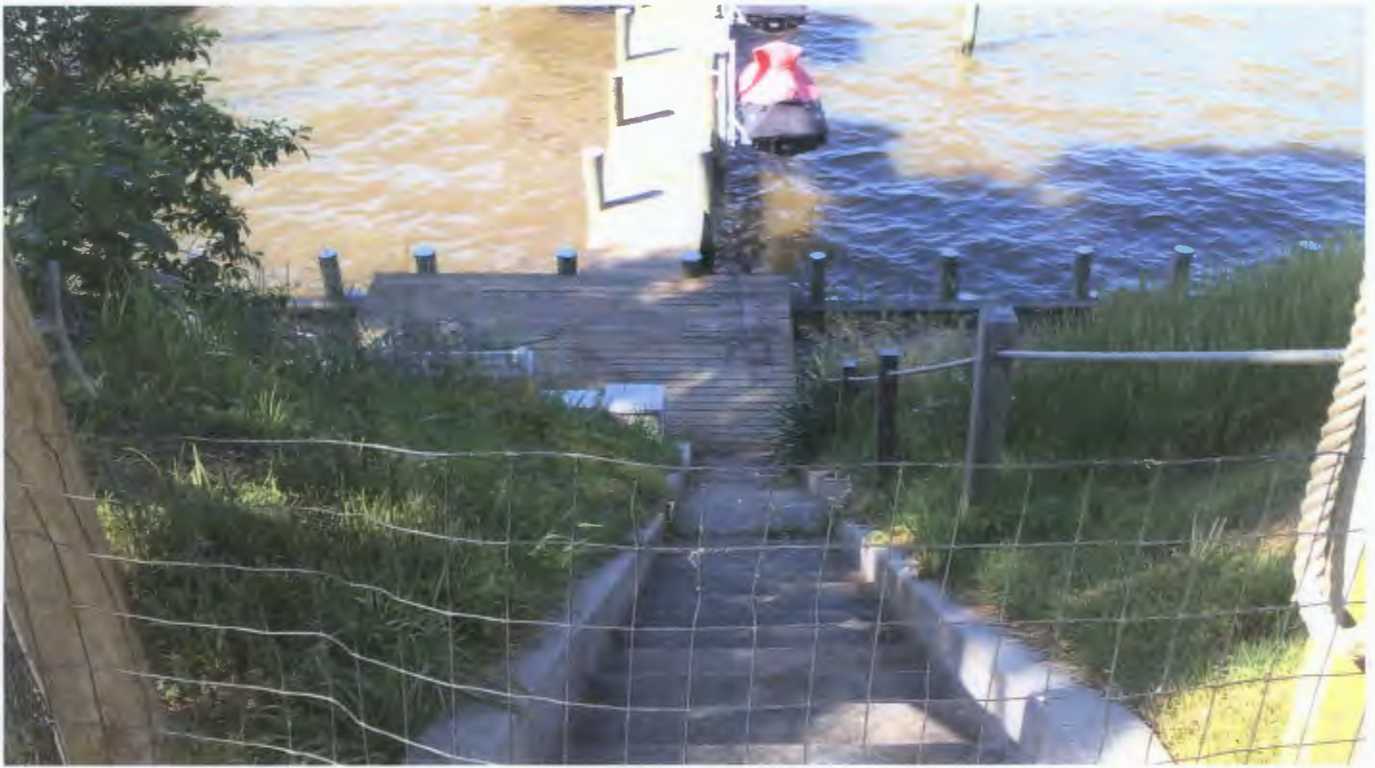
STANDING AT FRONT OF YARD FACING SOUTH
