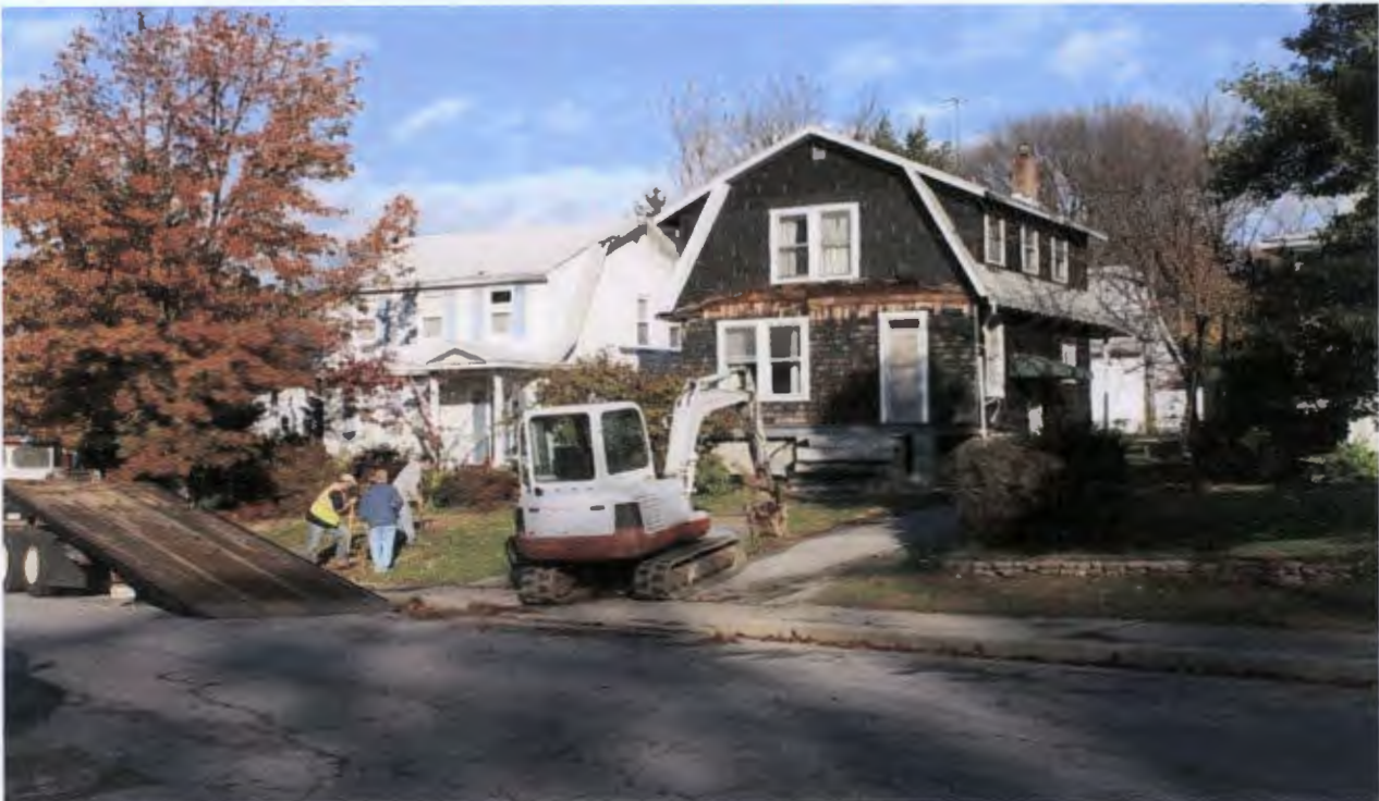
Photo 1: Structure at 802 Overbrook Road prior to demolition.
