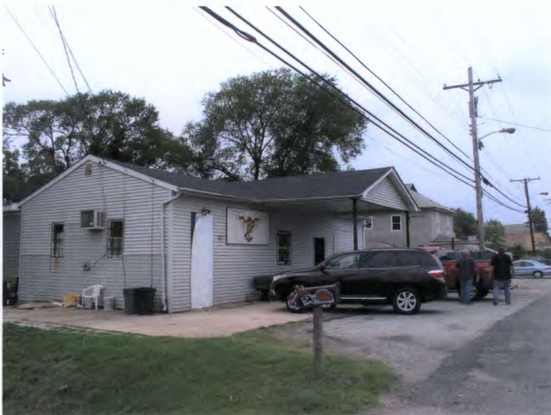
Front of existing building facing west along Sparrows Point Road
