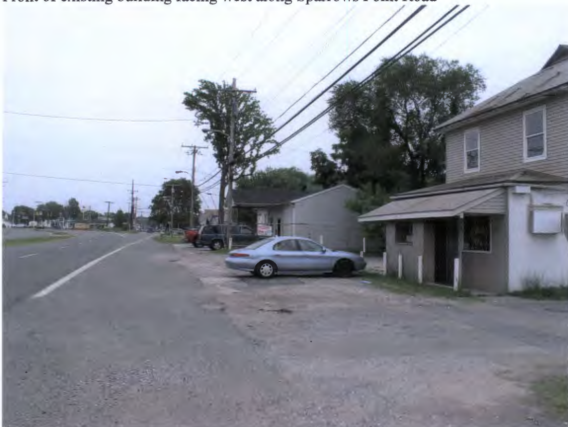
Front of adjacent building looking east toward subject site beyond
