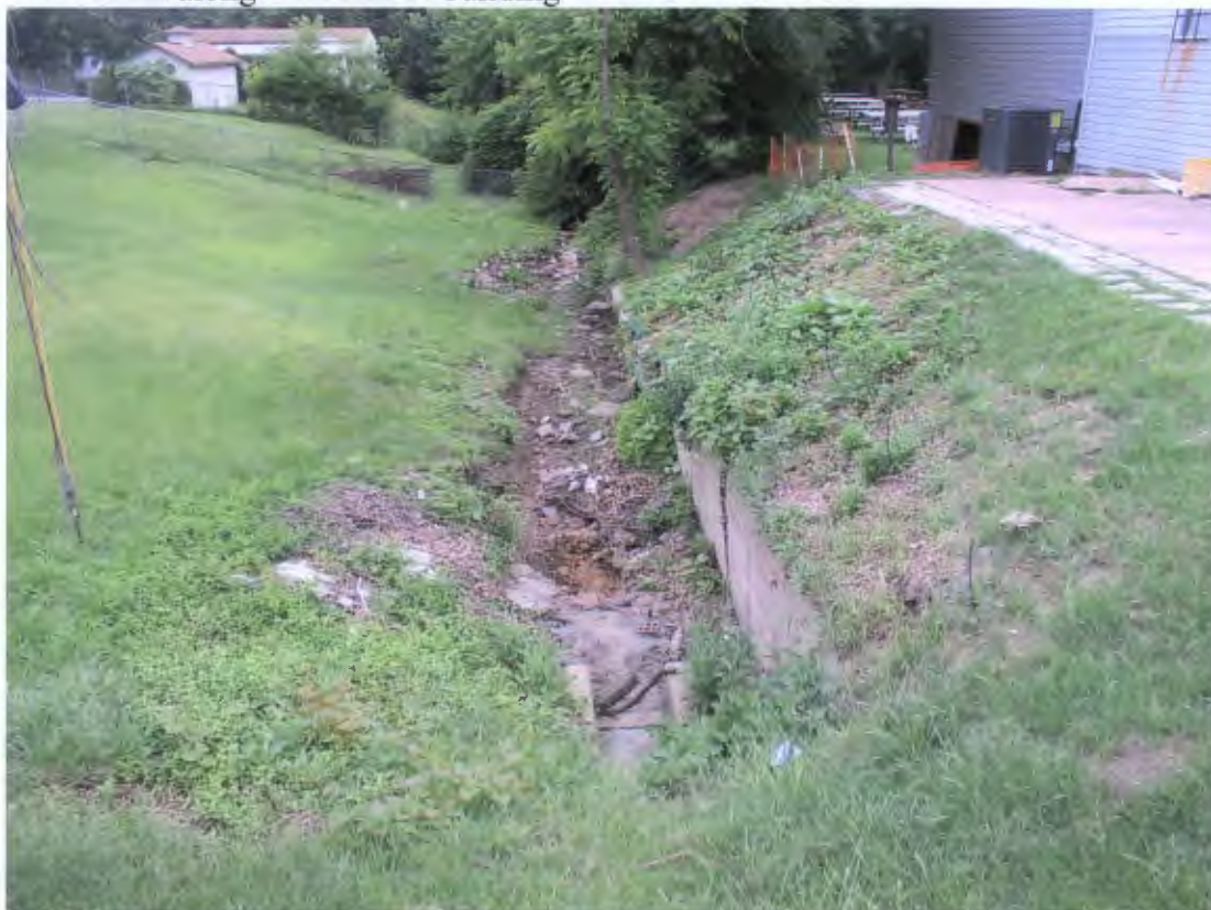
View south along east side of building
