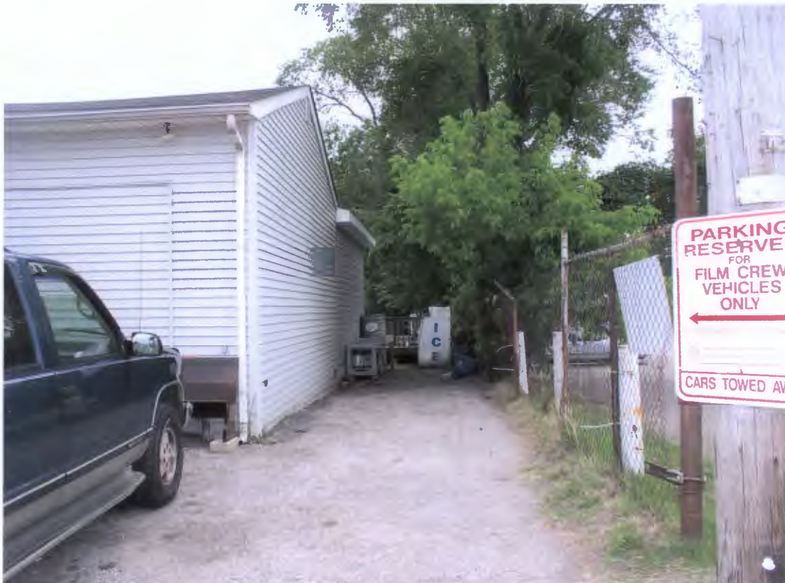
View south along west side of building
