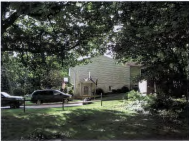
Additional side view of West side of property where proposed addition is to be built. (Photo taken from neighbor's lot.)
