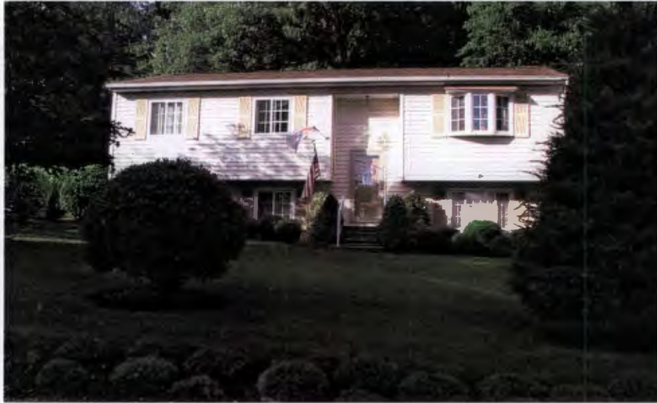
Front view from Mineral Avenue of existing house.
