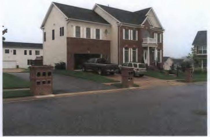
Coming down the street 2
