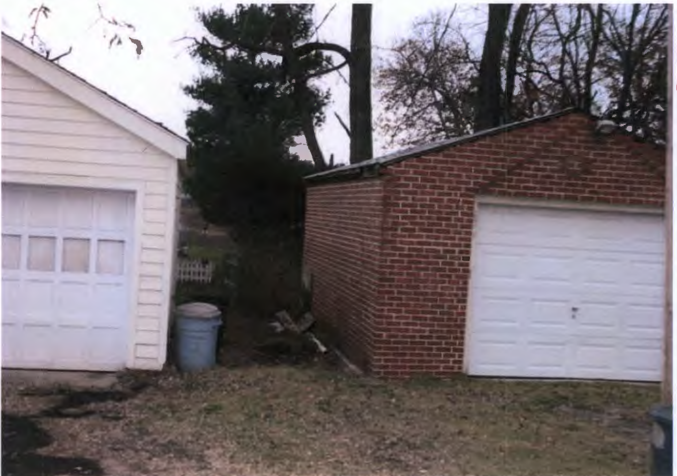
SITE EXISTING GARAGE
