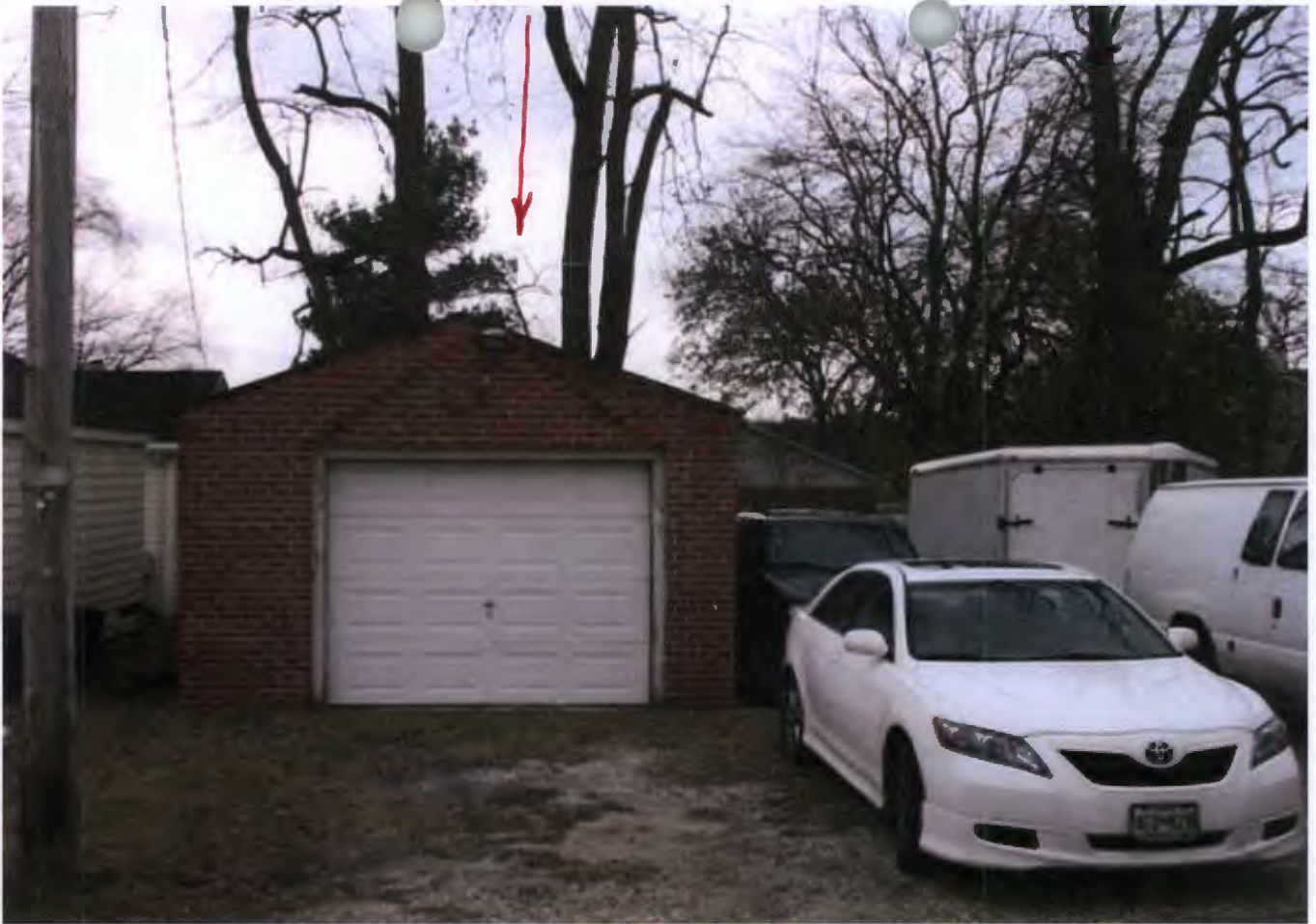
SITE - EXISTING GARAGE
