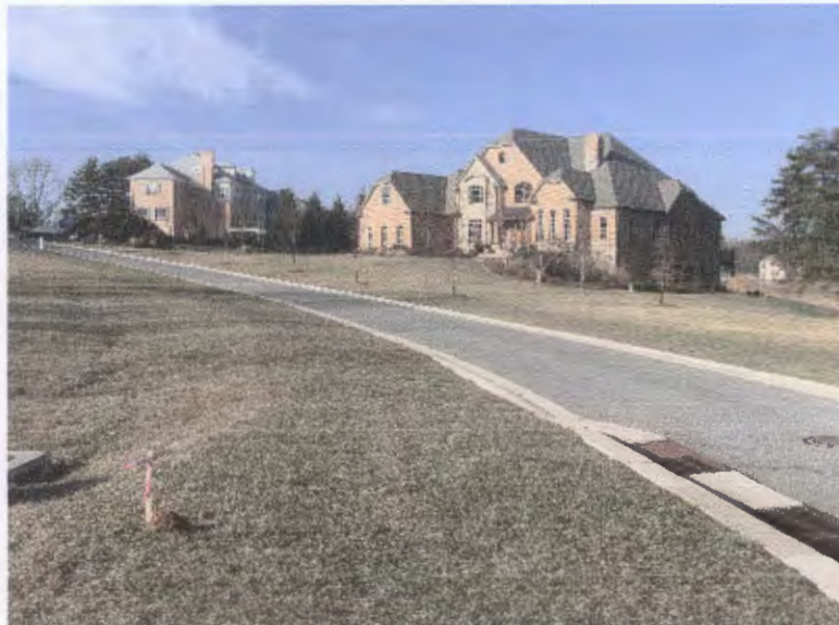
FROM NE CORNER LOOKING SOUTHWESTERLY ALONG STREET
