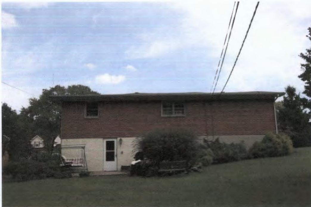
Photo 4 Rear of House (addition would be to right but further back (ie,towards front of house))
