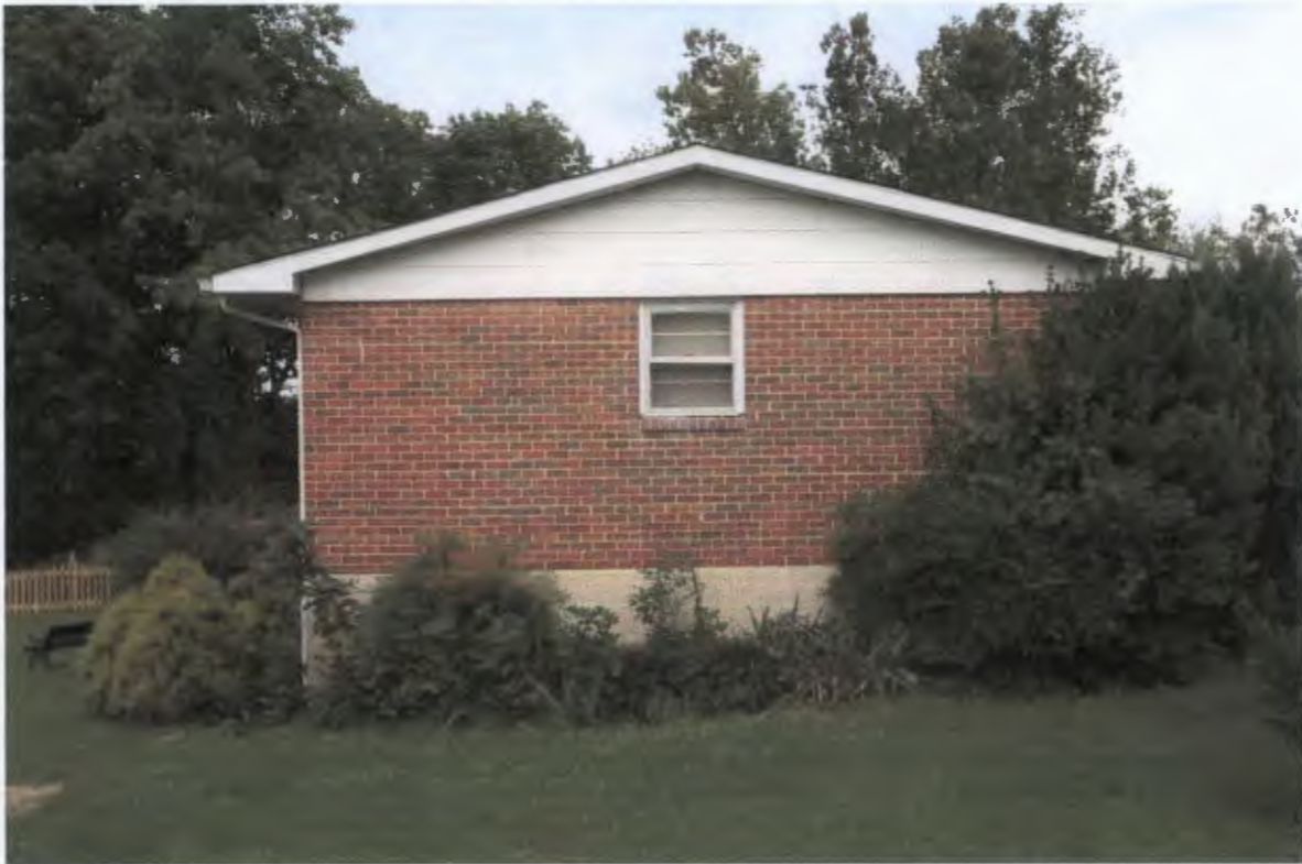
Photo 3 Left side of House where addition would be
