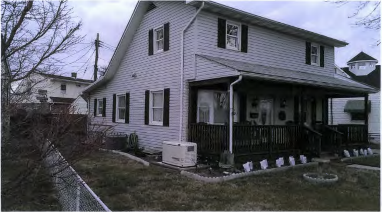
Front elevation of subject property (8257 Bullneck Road)
