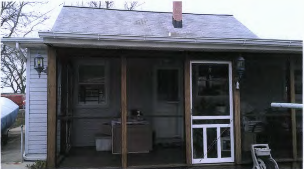
Rear elevation of subject property showing covered porch
