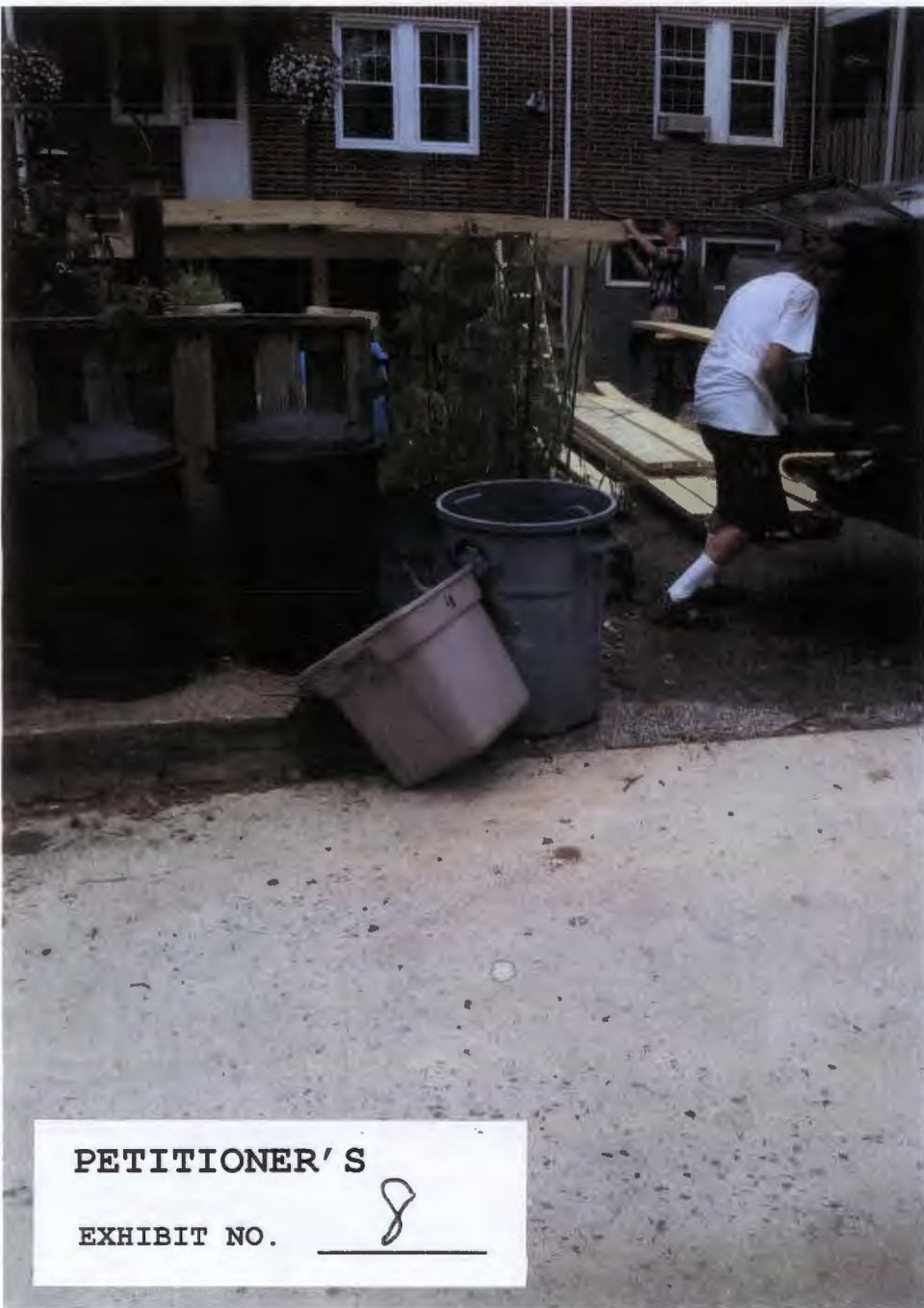
312 Hopkins Road - July 8, 2011 Construction
