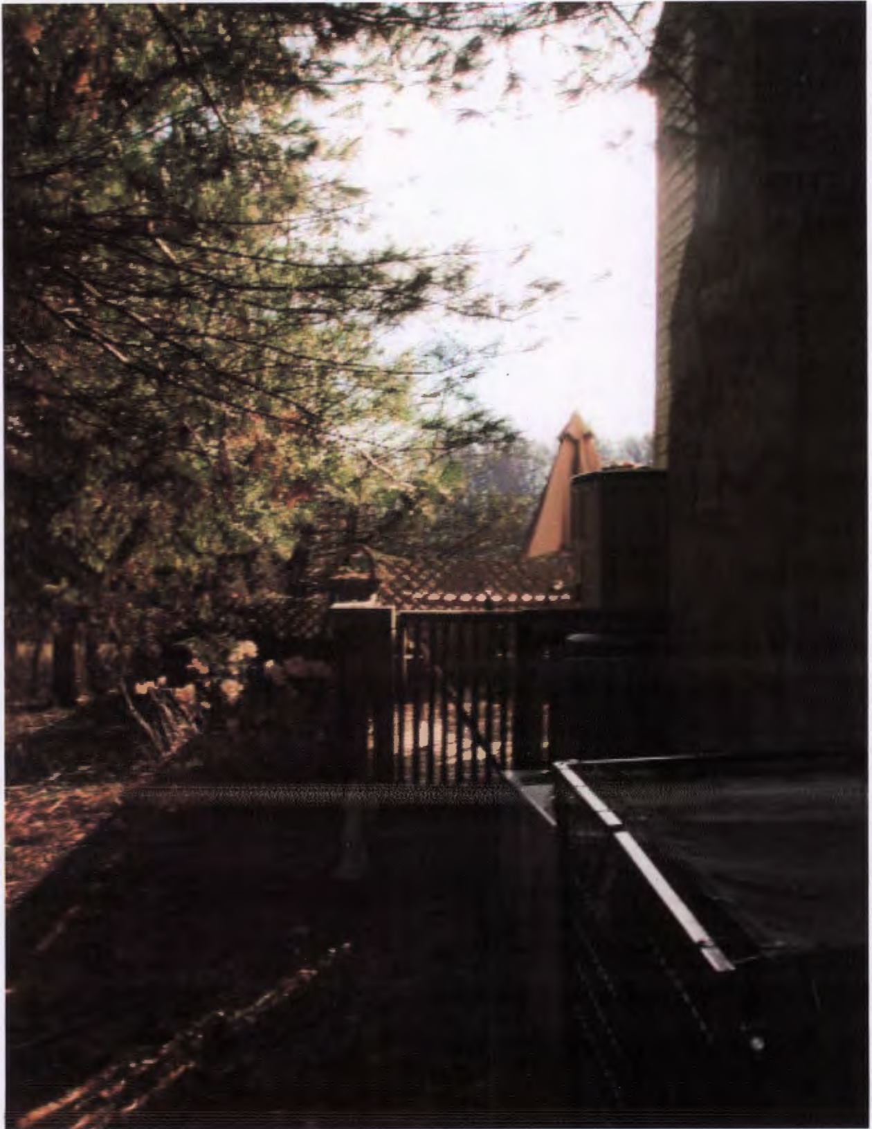
View of old deck from front left side of 11823 Manor Rd house
