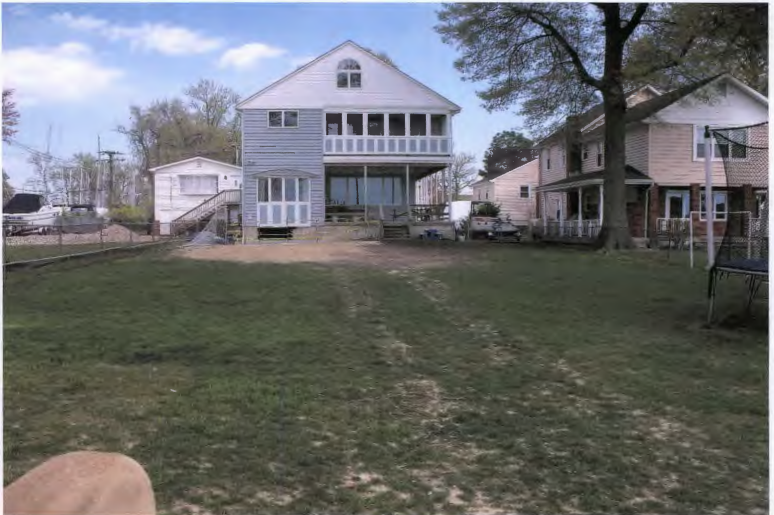
View of yard from bulkhead
