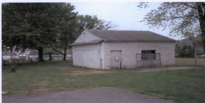
7815 GARAGE TO BE REPLACED
