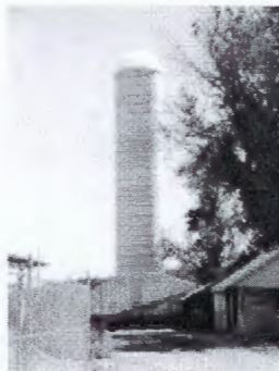
"20' x 108' Tower in NJ" With Antennas Hidden Under the RF Friendly Roof.
