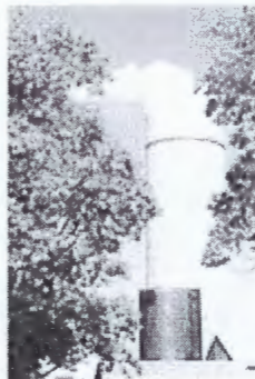
"The Old and the New" Who would believe that the new, taller silo was built to house antennas and equipment for multiple carriers?
