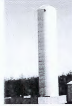
"Silo For A Cell Tower" 20' x 100' Antennas Hidden Near The Top LOCATED IN NORTHERN VA
