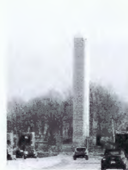
"20' x 140' Beside The PA Turnpike" With Antennas Hidden Under The RF Friendly Roof.
