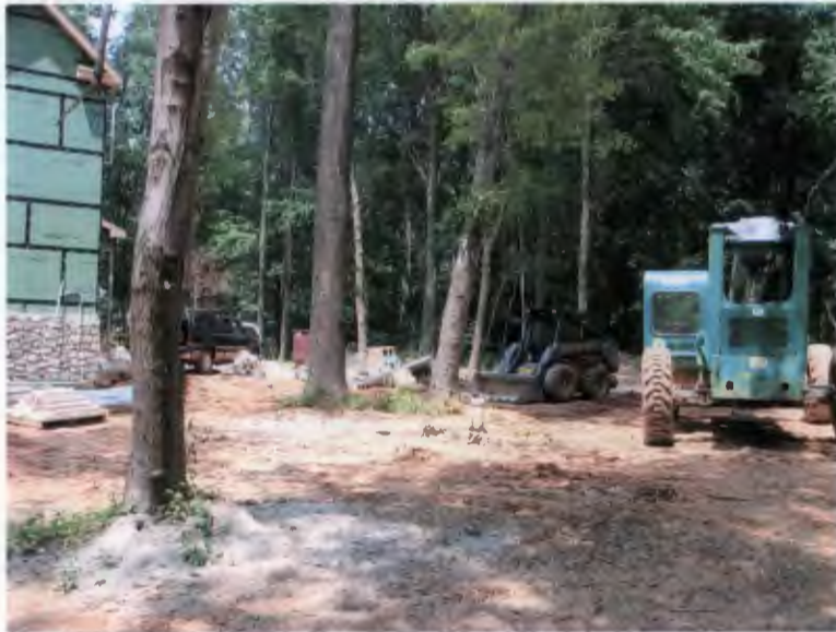
15 – View from court toward 27 Mansel Circle
