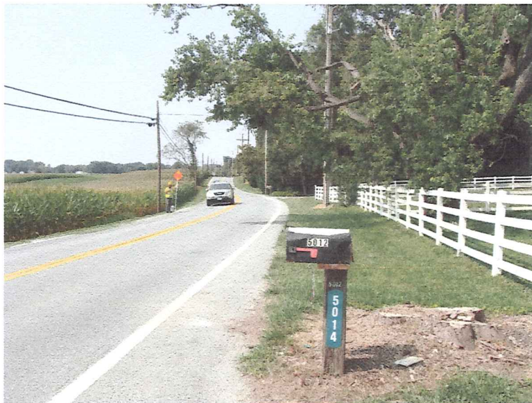
LOOKING SOUTHWESTERLY ALONG MT. CARMEL ROAD
