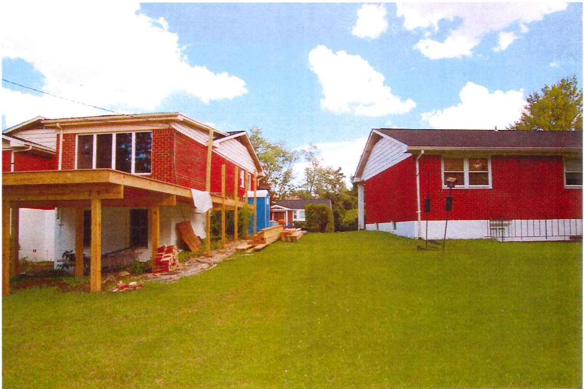
Photos of the 18' x 19' deck with 4' wide walkway between the deck and existing side porch / kitchen door that is currently under construction (Permit # B-792036, issued 7/2/2012). The walkway will not be completed and/or tied into the side porch until a decision is returned by the County on the side setback variance request.
