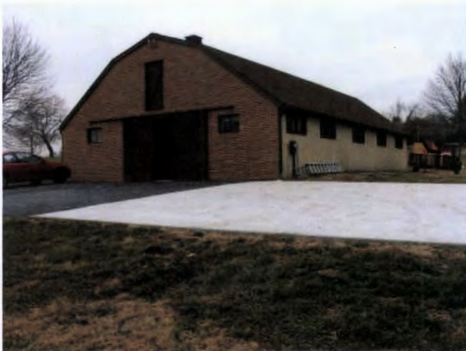
U - FRONT (SOUTHWEST) ELEVATION OF BARN #2 (17'+/- HIGH)
