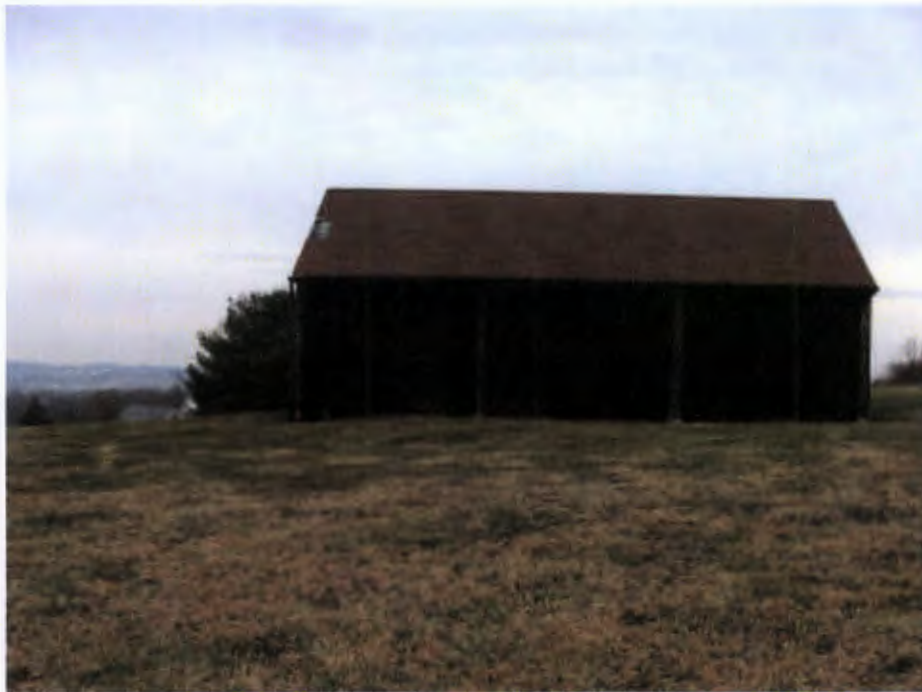
P - EAST ELEVATION OF EXISTING BARN #1 (17'+/- HIGH) (#13101 IS VISIBLE OVER THE HILL TO THE LEFT OF THE BARN)
