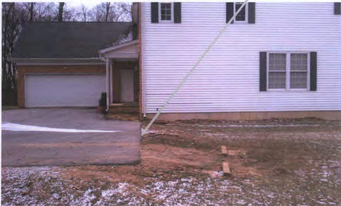
View F) from front west corner of garage addition, pointing east, showing west face of house and front line of house and driveway rear edge. Front east garage addition corner is marked
