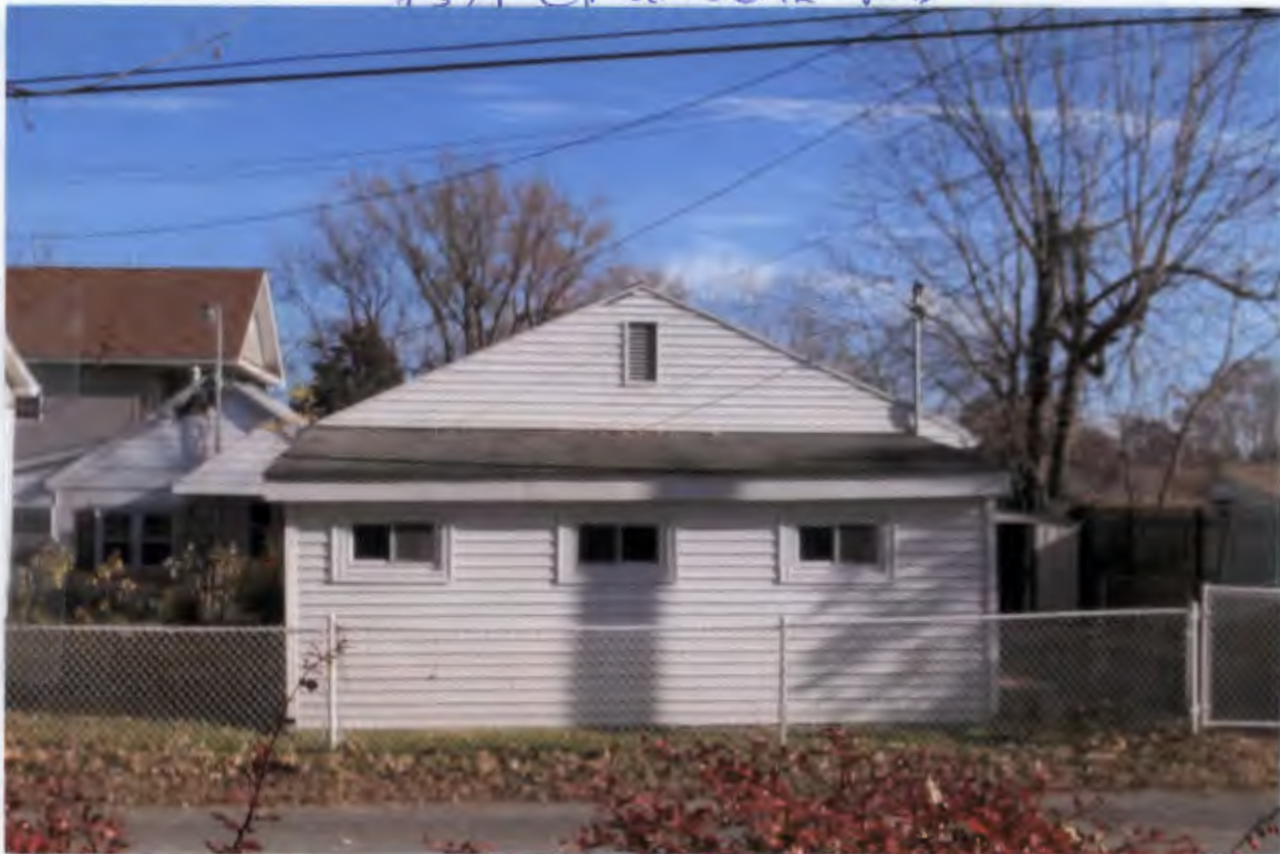
Side view of in law suite view from Patapsco Rd Pet No 4 7321 Greenbank Rd
