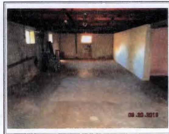
BASEMENT - UNFINISHED AREA
