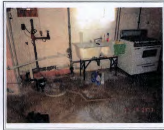
BASEMENT UTILITY AREA
