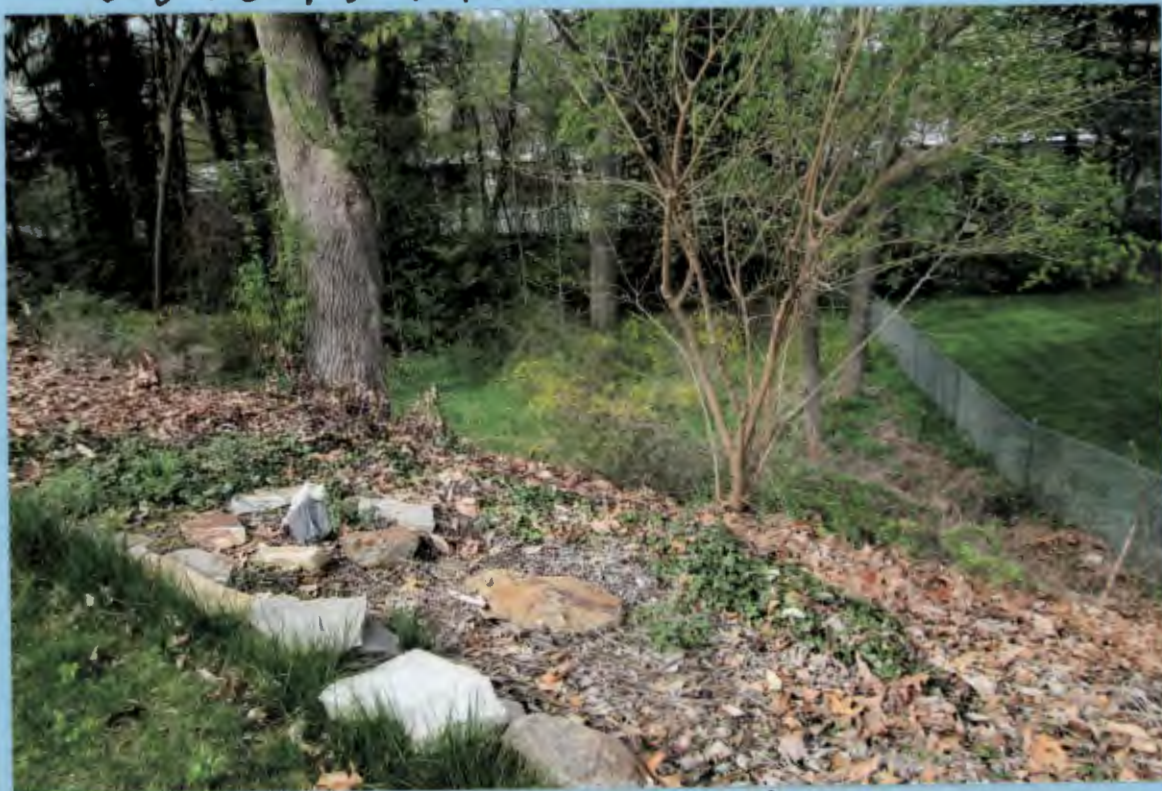
Large Slope From Behind Parking Pad 608 Fence divides 608 from 604 - (Belongs to 604)
