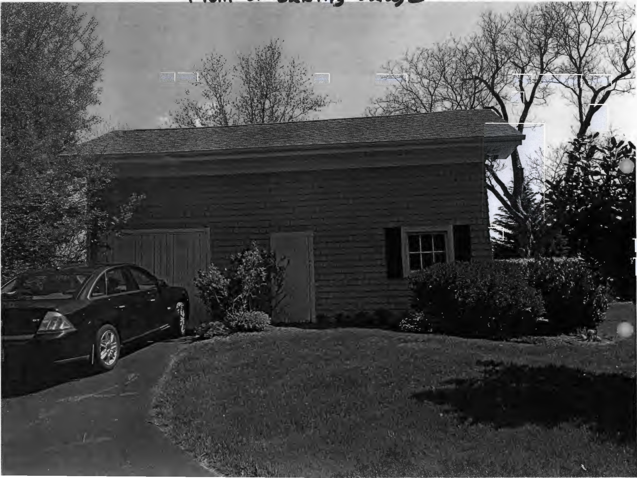
Front of Existing Garage
