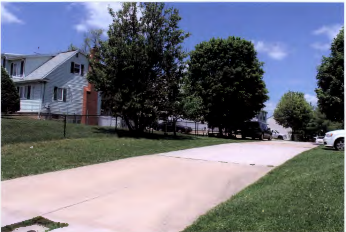
SIDE YARD & COMMON DRIVEWAY OF HOUSES TO REAR.
