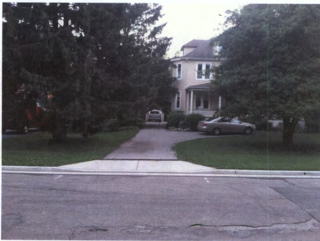
VIEW OF 9 N BEAUMONT FROM STREET
