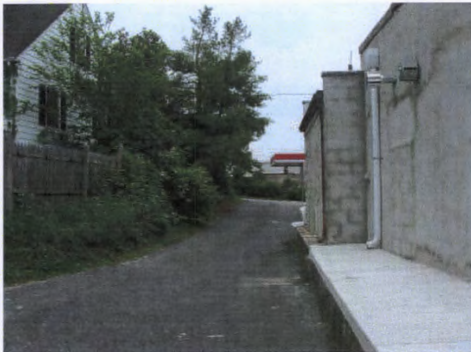
L – REAR OF BUILDING LOOKING TOWARDS LINWOOD AVENUE
