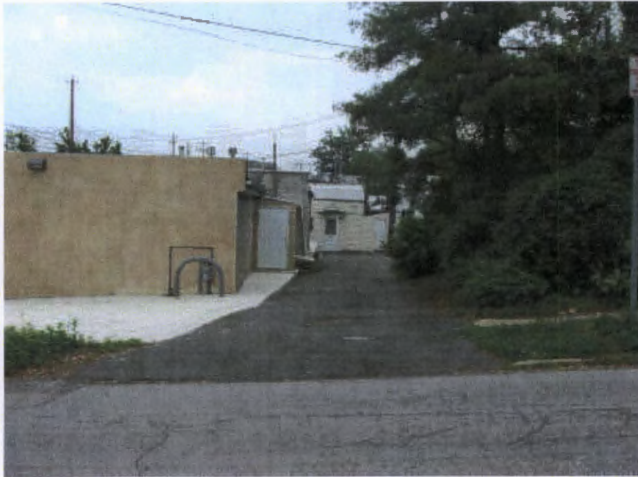
C – VIEW ALONG REAR OF BUILDING, LOOKING SOUTHWESTERLY
