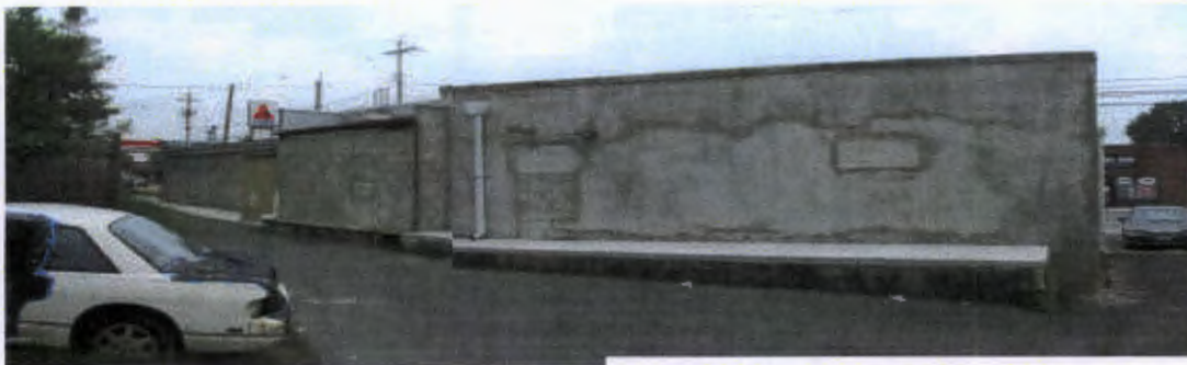
D – REAR OF BUILDING
