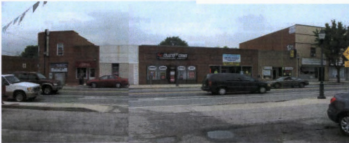
M – STOREFRONTS ALONG EAST SIDE OF HARFORD ROAD
