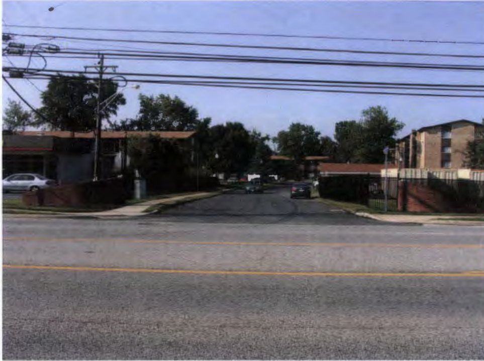
C – ENTRANCE TO SITE – FOXCLIFF COURT
