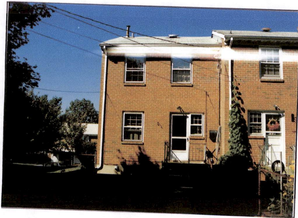
REAR OF SUBJECT PROPERTY
