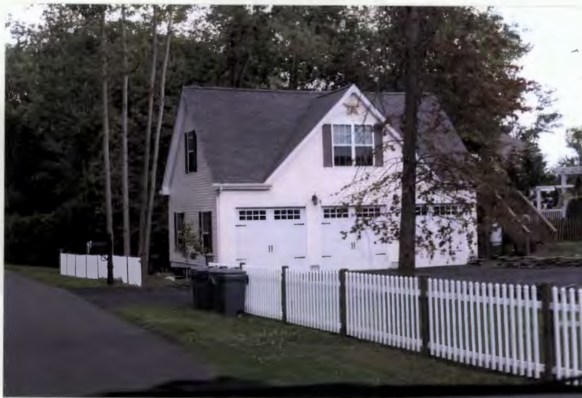
11315 Beach Rd ↑ 25ft set back at Road 100 feet west of subject Property
