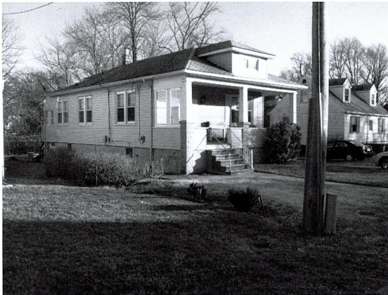
SOUTHWEST SIDE VIEW OF THE PROPERTY
