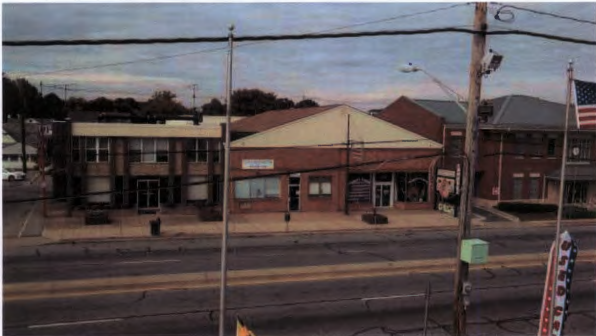
Northeast of Site
