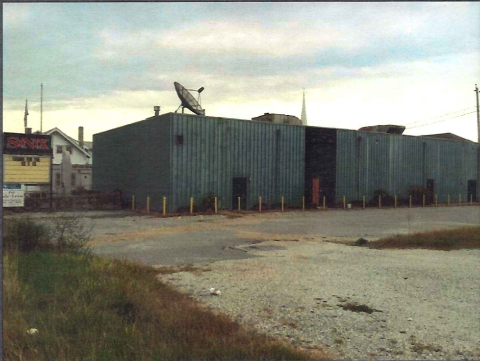
Looking North at Existing Building
