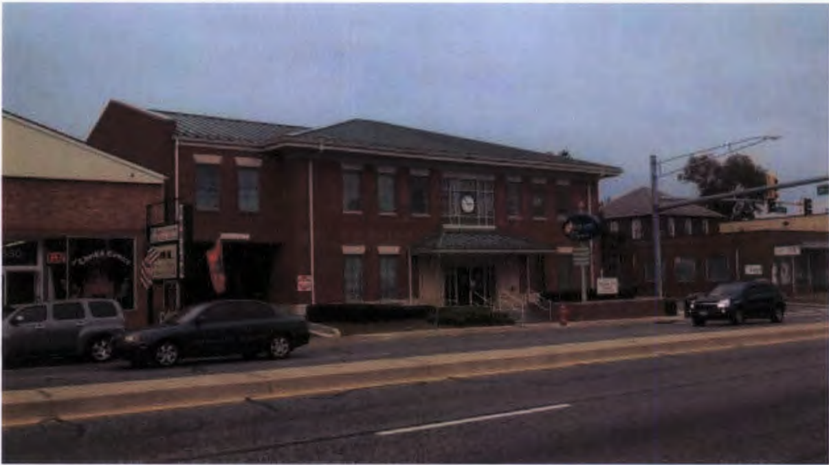
Northeast of site on north side of Eastern Boulevard
