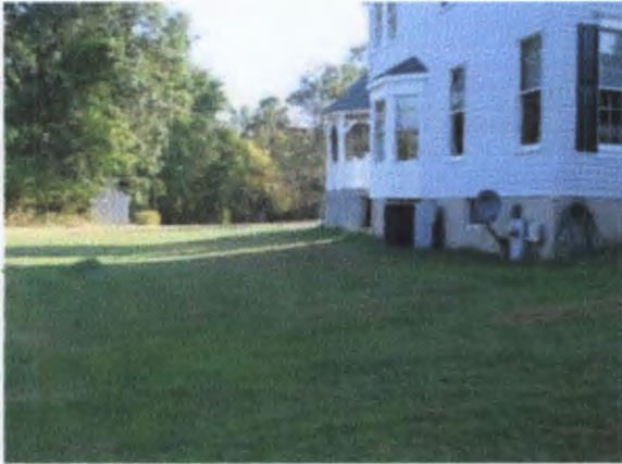
Figure 6: Buried Electrical Service West Side Of House
