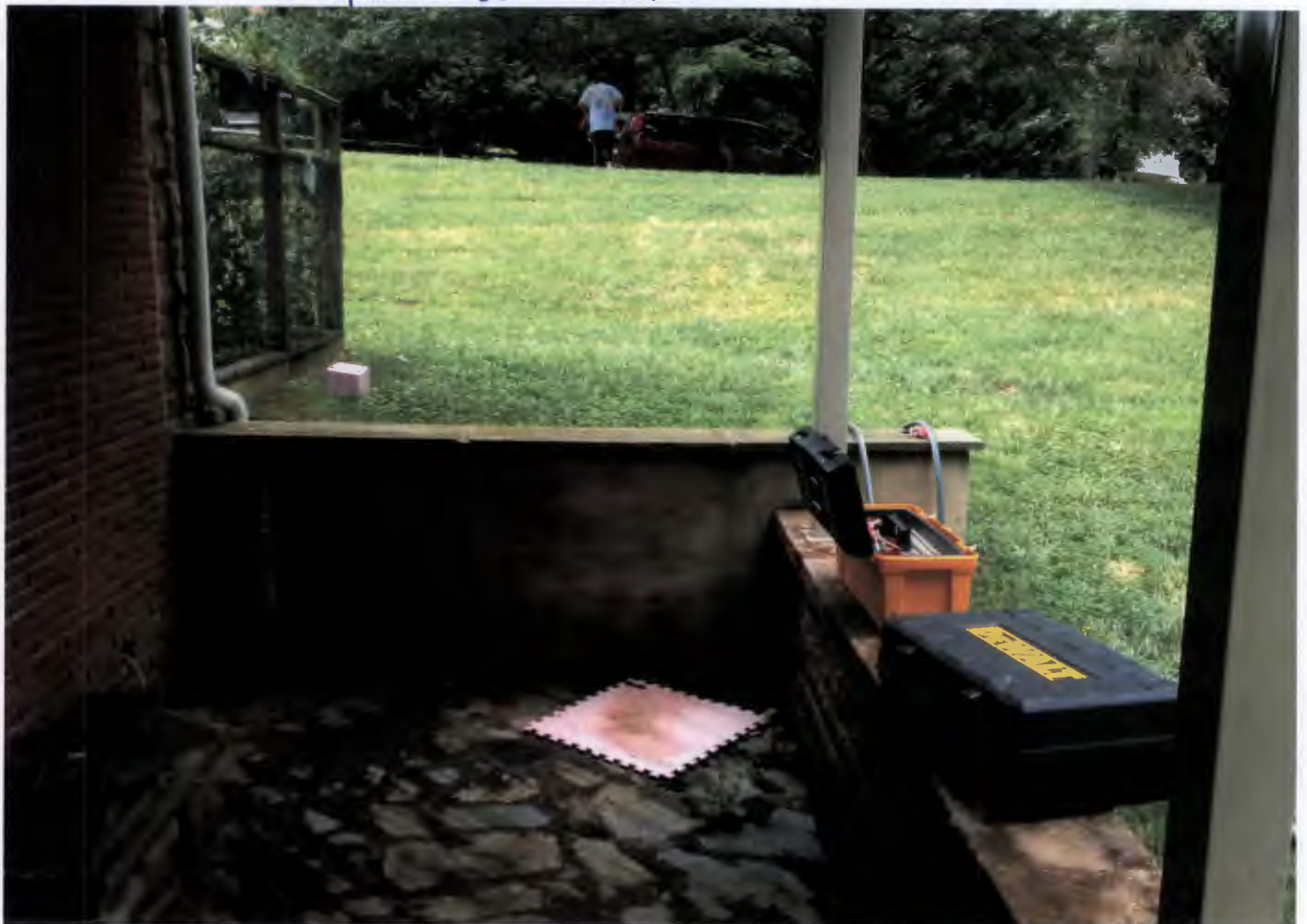
under deck looking left to Benton Road
