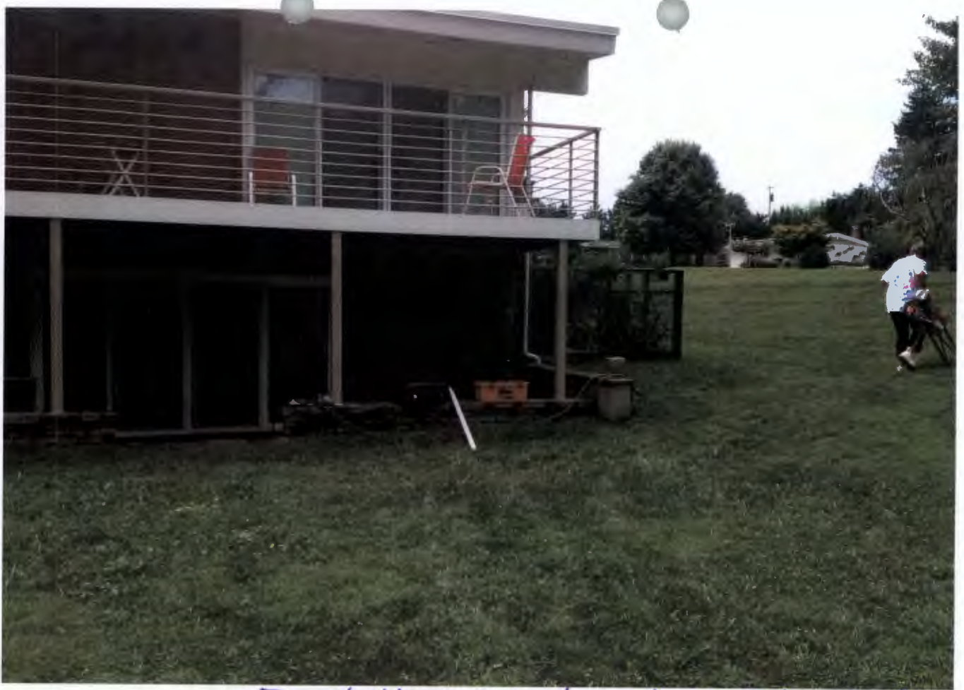
From Yard looking to deck - Bendon Rd. side →
