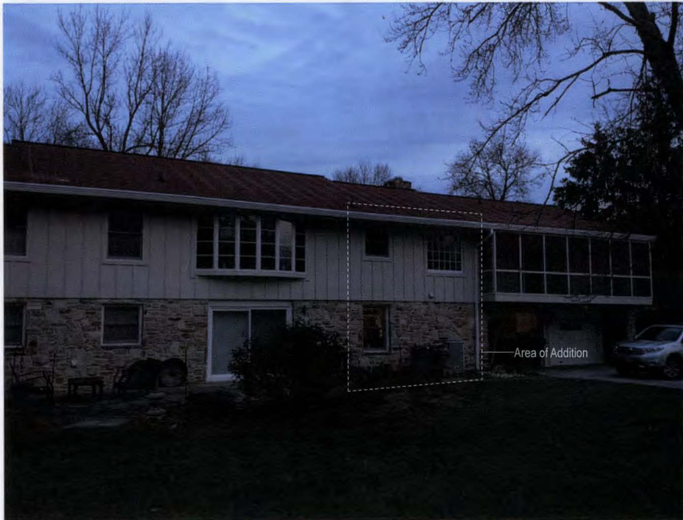
View from rear yard looking north Existing house photographs 3 of 5
