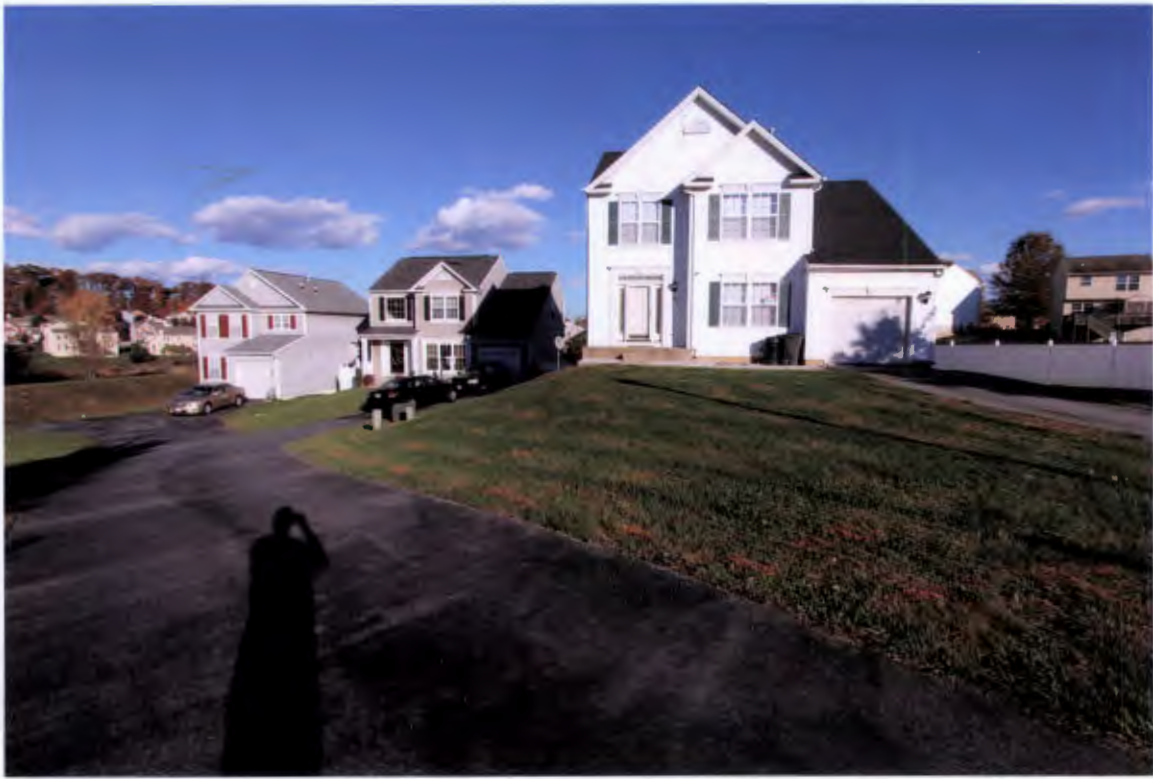
FRONTAL VIEW OF 30, 28, AND 26 CLEMATIS COURT
