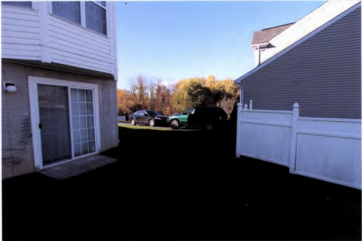
REAR VIEW OF AREA FOR ADMINISTRATIVE VARIANCE
