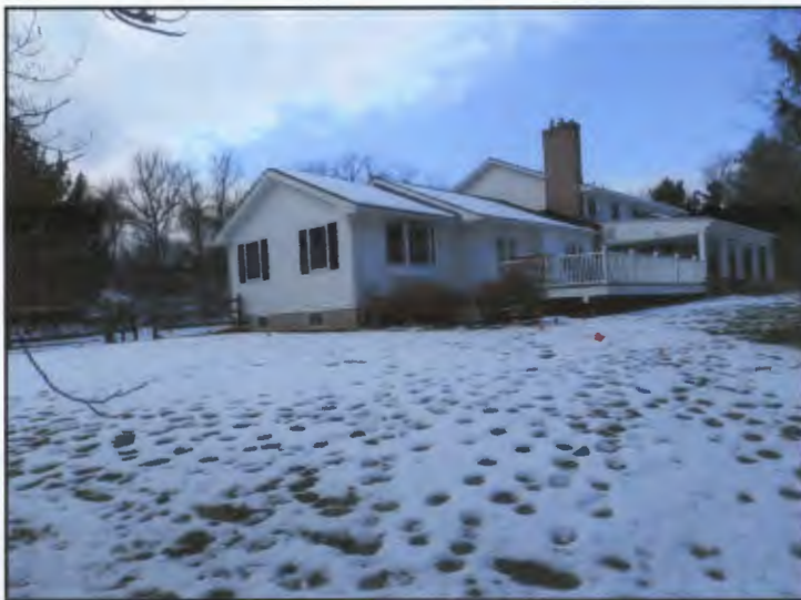
From Rear Corner of Lot 1200 Cowpens Avenue
