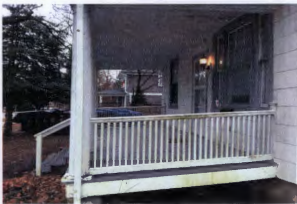
View of adjacent property.
