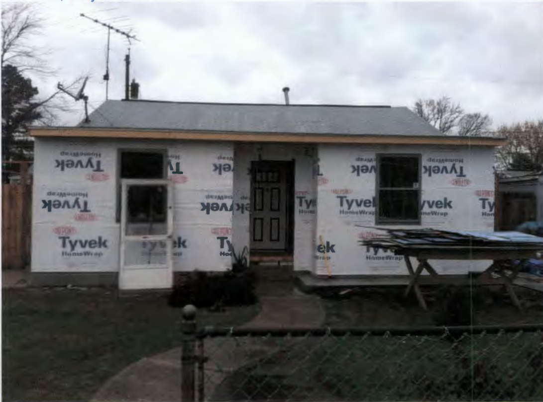
Enclosing front porch
