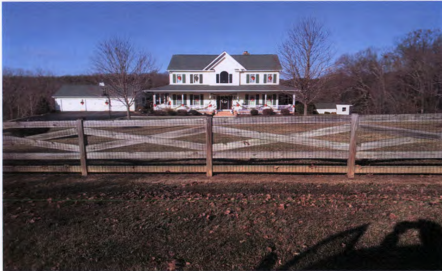
Photo 3: Larger dwelling east of 6200 Glen Falls
