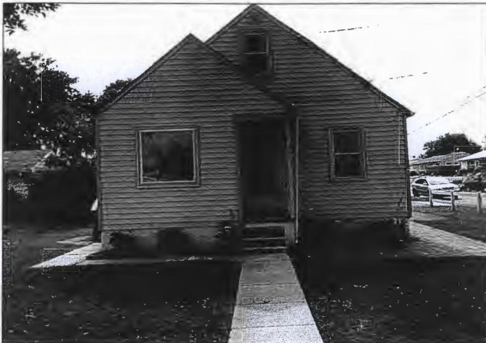
Front View of Subject - Facing Old Harford Road
