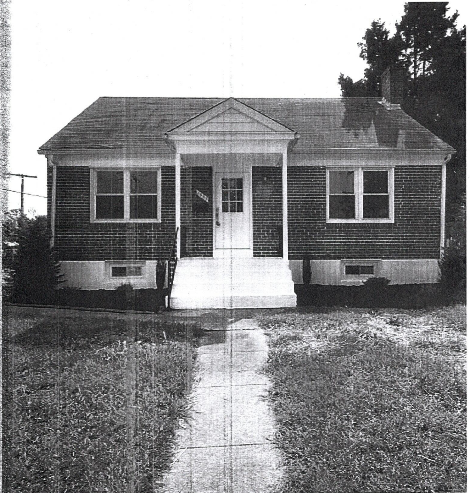
Front View of Dwelling
