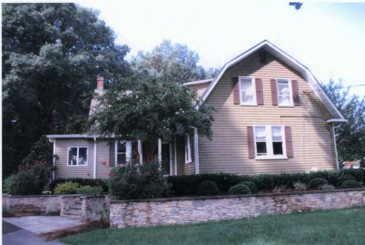
Picture of the front of the house
