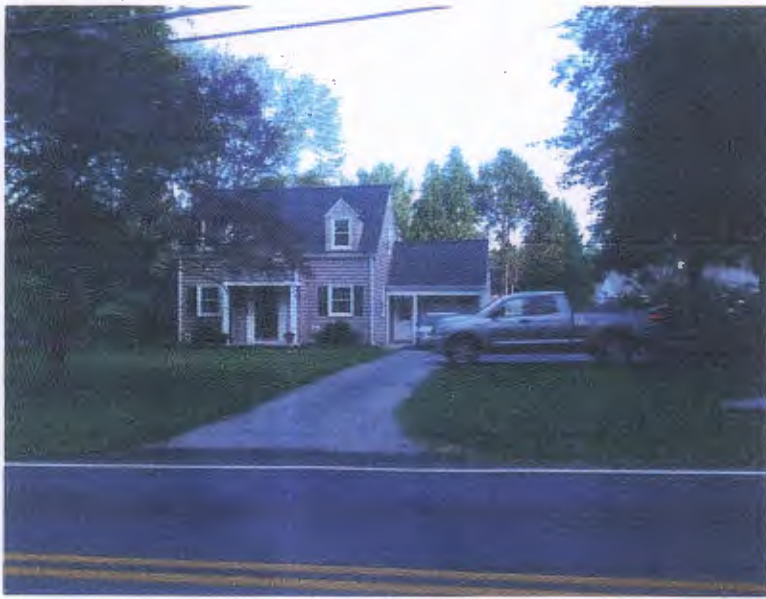
FRONT VIEW FROM PROVIDENCE RD.
