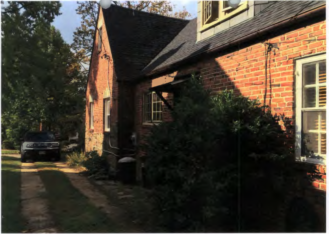
LOOKING FROM REAR OF HOUSE
